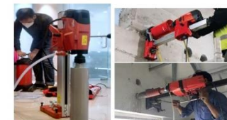
23. Diamond Core Cutting Machine for measuring current strength (Destructive Test)
